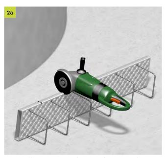
For round formwork, depending on the formwork radius, make several cuts with uniform spacing using an abrasive cutter on the side walls on both sides of the casing.
