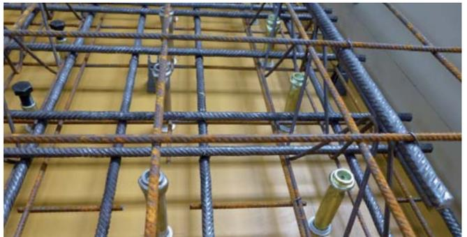
FIXING OF PROPS ON PRECAST ELEMENTS
